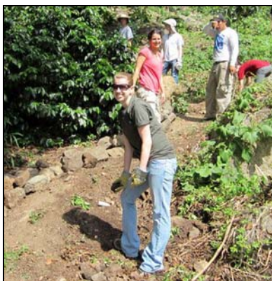
Rebuilding a washed-out trail at La Atitlàn.
